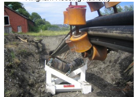
Peddocks Island Utility Installation
